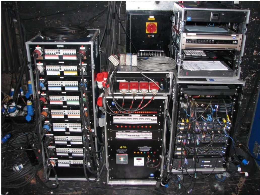
*Mains distribution equipment backstage. The rack on the left is a 108 x 10 Amp channels of single phase power distribution, in the centre is a 16 way three-phase distribution unit, the rack on the right is control data distribution.*
