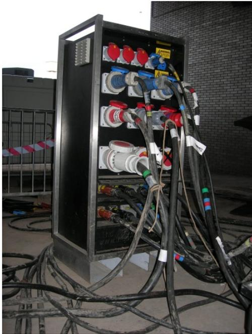
*A typical mains distribution unit. Along the bottom can be seen the single-pole connectors, each rated for 400A. There is a supply in and a loop-through to the next distribution unit. The outputs are a variety of BS EN 60309 ('ceeform' type) connectors in single and three phase, ranging from 16A to 125A. The protective devices are at the rear of the unit, and it sits on metal skids so can easily be transported using a forklift or similar.*
